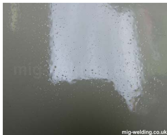
Overspray of finished surface
